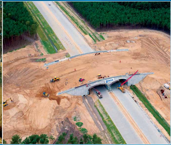
SuperCor® corrugated plate structures in the WD-3c animal overpass
