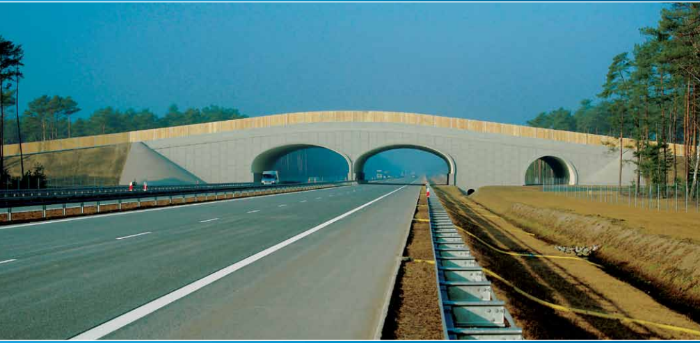
SuperCor® corrugated plate structures and ViaWall A type 1 MSE walls in the WD-69a animal overpass
