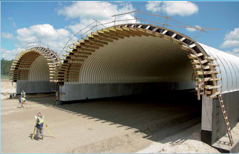
SuperCor® corrugated plate structures in the WD-63a animal overpass
