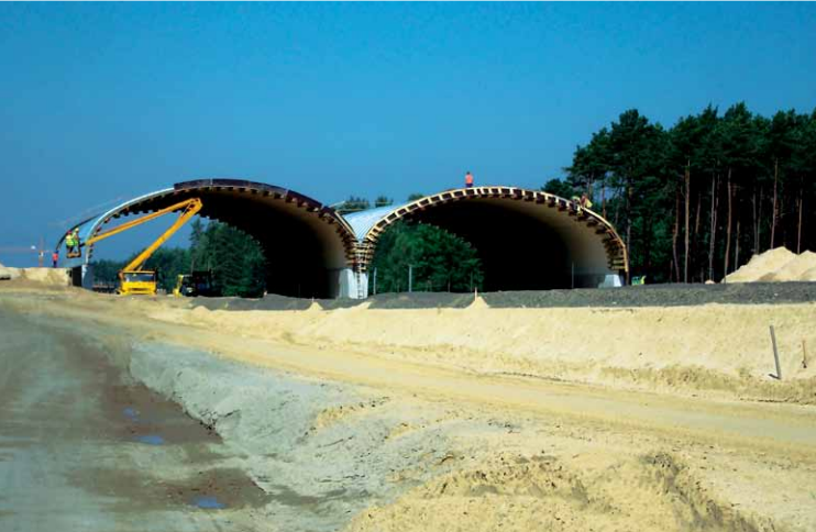
Assembly of SuperCor® corrugated plate structure in the WD-69a animal overpass
