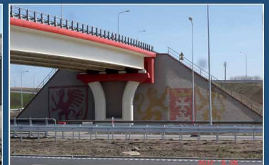
ViaBlock retaining walls
