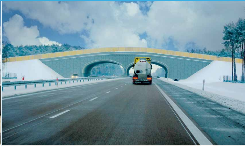
SuperCor® corrugated plate structures in the WD-3a animal overpass
