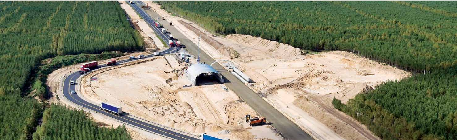
Assembly of SuperCor® corrugated plate structure in the WD-10a animal overpass
