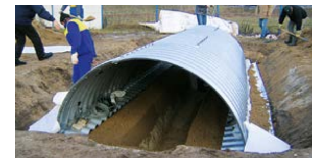
Fot. 3. Connection of MultiPlate MP200 structure with flexible footing
