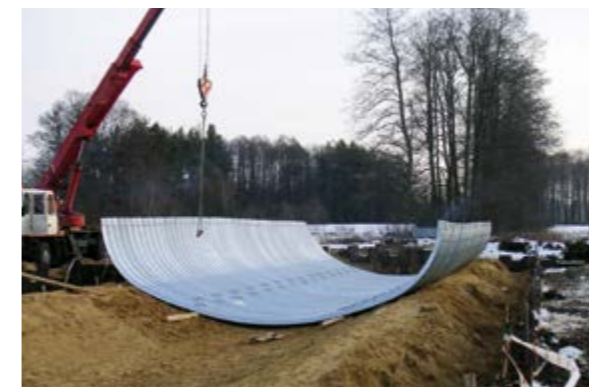
Fig. 11. Connection of SuperCor® structure with flexible footing
