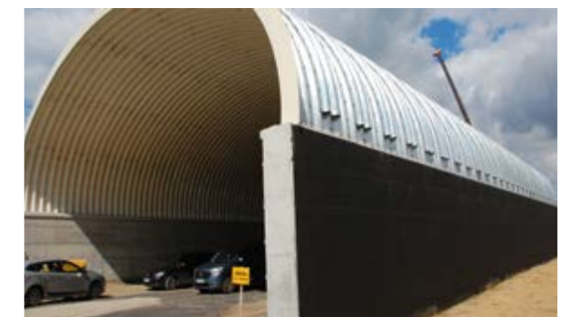
Fig. 9. Placement of the ribs in longitudinal direction of the structure
